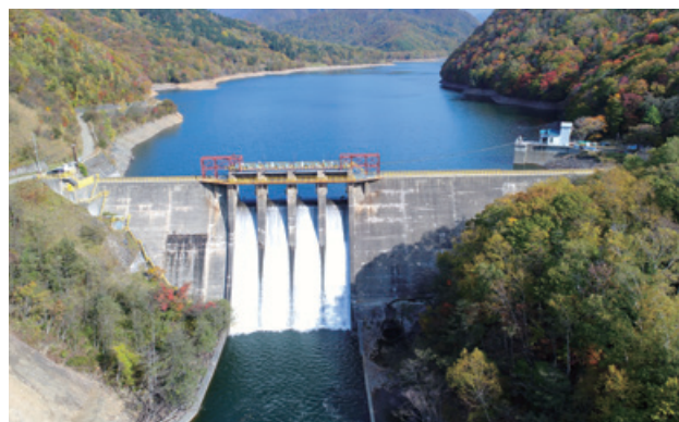
No. 3 Power Plant Dam
