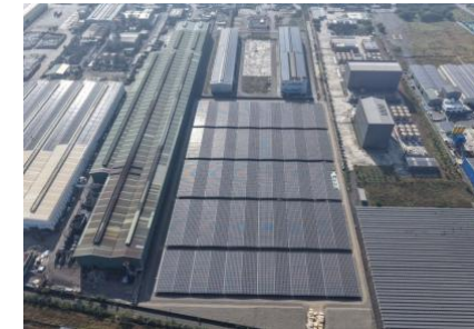
Solar power generation system
