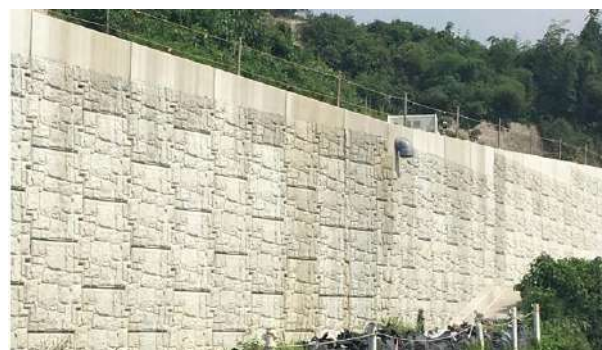
External view of the Terre Armée method
