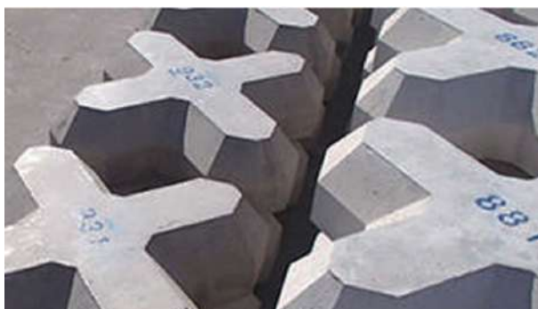
Wave-dissipating and foot protection block
