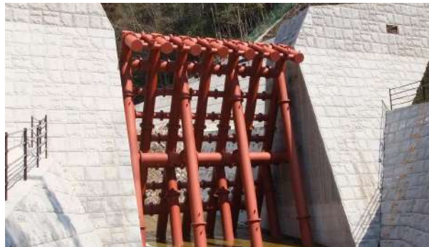
Permeable steel slit dams
