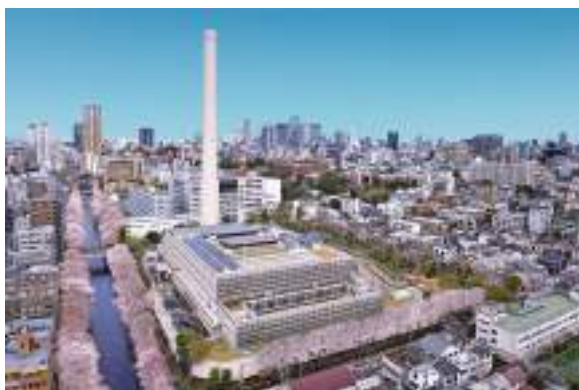
Waste-to-energy power generation plant
