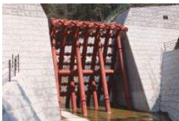
Permeable steel slit dams
