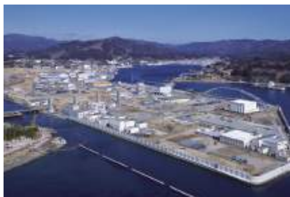
Hybrid tide embankments
