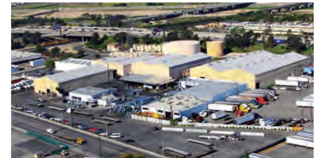
Main plant at CEMCO
