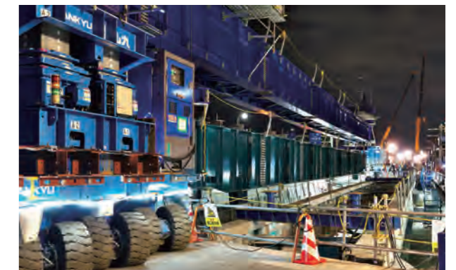
Bridge replacement work at night
