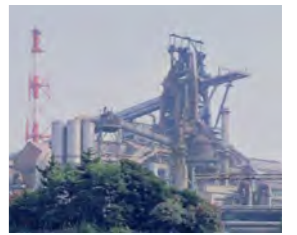
Chiba No. 6 blast furnace
