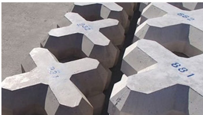
Breakwater armor block
