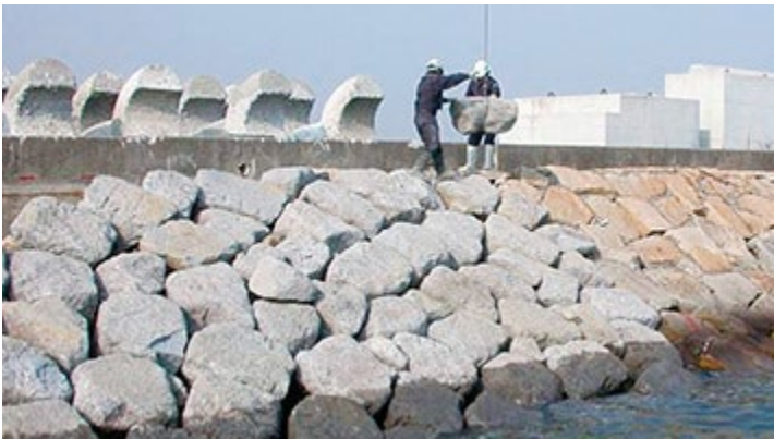
Coastal construction work using artificial stones made from steel slag hydrated matrix
