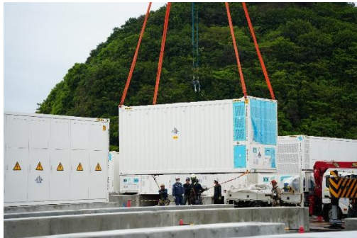
Delivery and installation of major equipment at the Shizuoka Kikugawa Power Storage Plant
