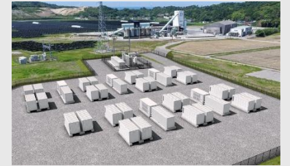
Image of completed Shizuoka Kikugawa Power Storage Plant
