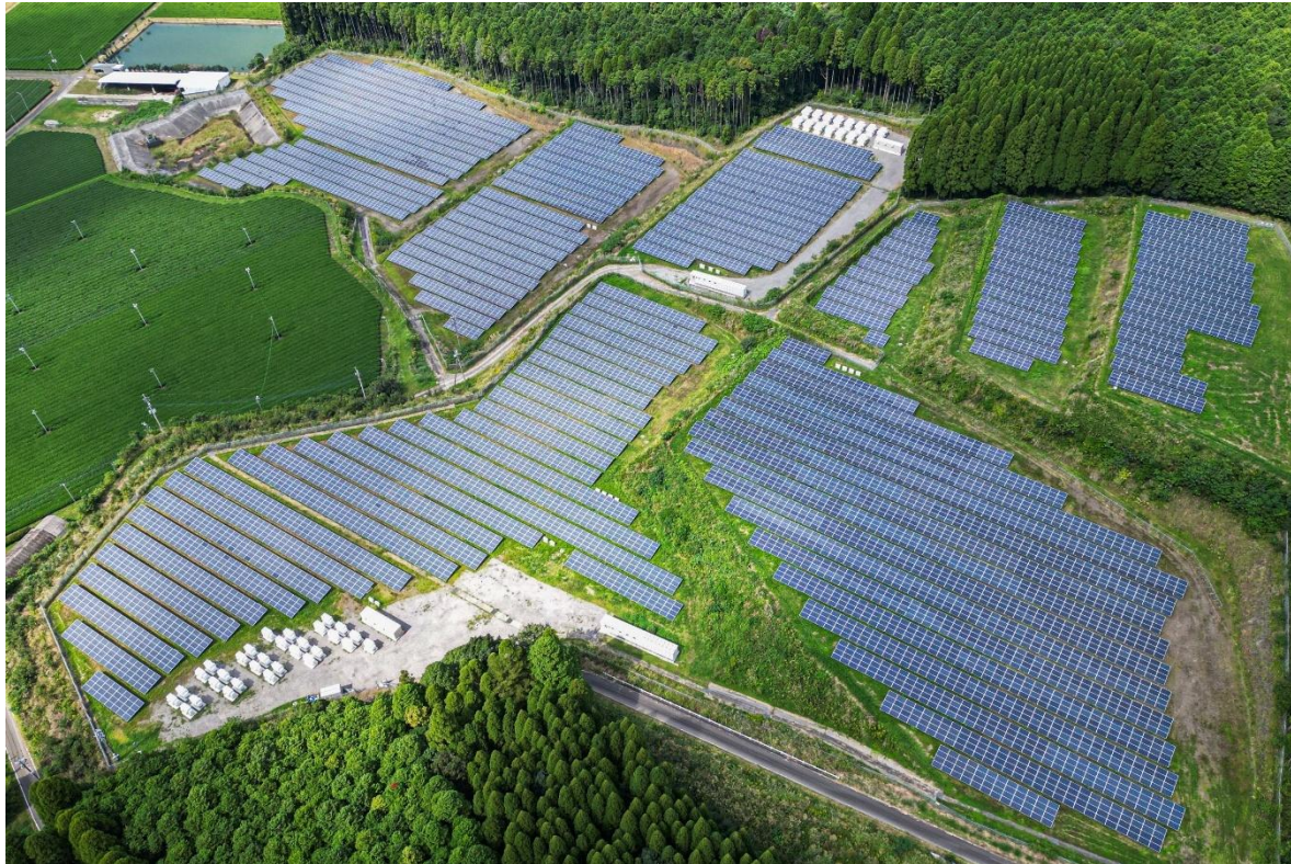
Solar power plant with co-location of storage batteries (located at Yusui-cho, Aira-gun, Kagoshima Prefecture)
