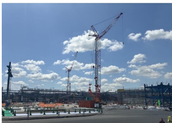
Large pilot facility under construction
