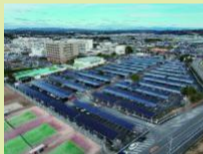
Solar carports established on the Kiyotake Campus of the University of Miyazaki
