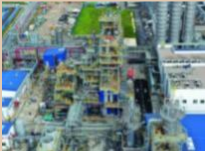
Second SPS facility that started commercial operation
