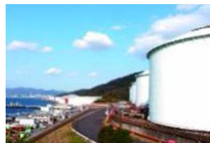
LPG tanks at the Tokumaya Complex
