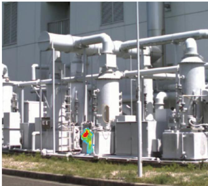
Gas monitoring solution makes gas leaks visible
