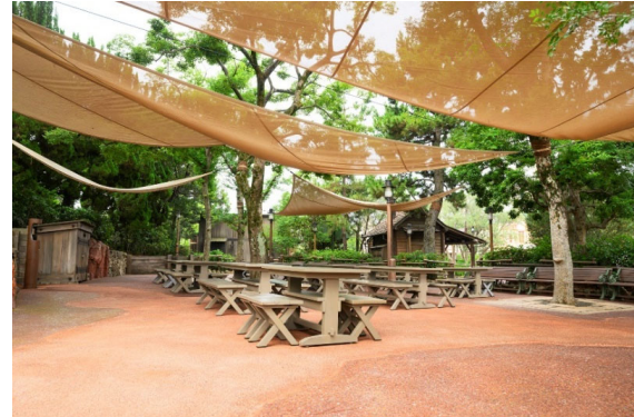
Tarps and water-retaining coating
