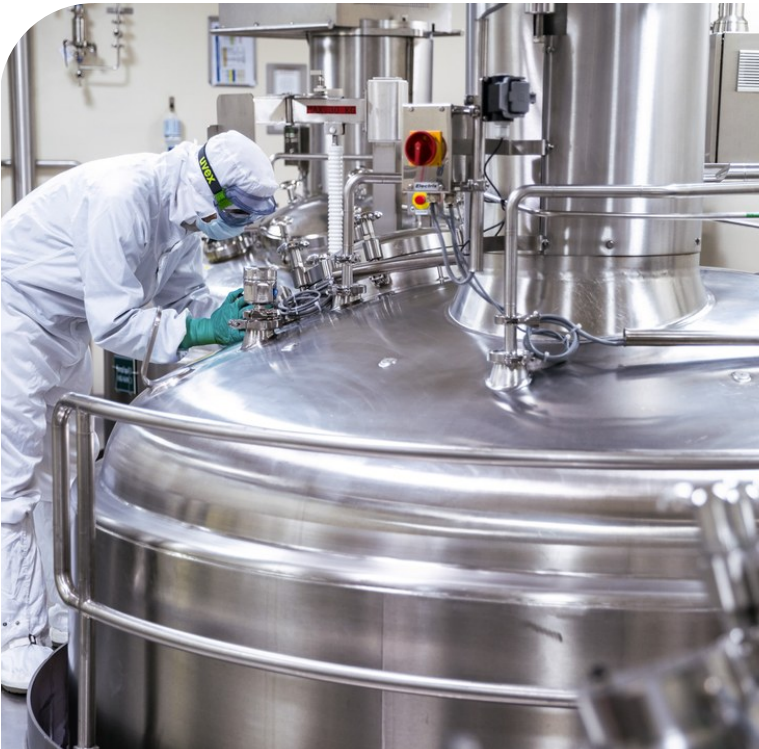
Our water recycling system in Lessines, Belgium, enables us to reuse 90% of our wastewater for an annual savings of 600,000 m³ of water – the equivalent water consumption of 18,000 people in Belgium annually.
