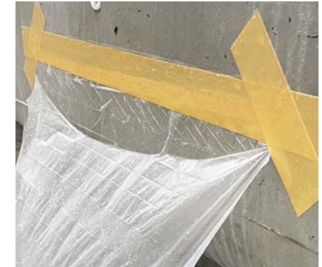
Temporary securing sheets or marking on a wet concrete surface
