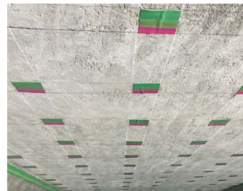
Concrete reinforcement method featuring fiber sheets affixed in a grid pattern
