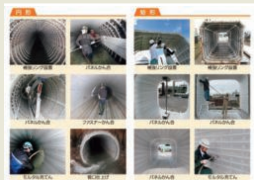
Construction examples using the pipe renewal method
