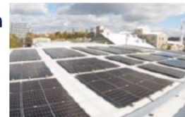
Solar system installed on highly durable waterproof sheet
