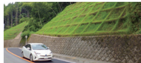
Slope constructed using the GT frame®
