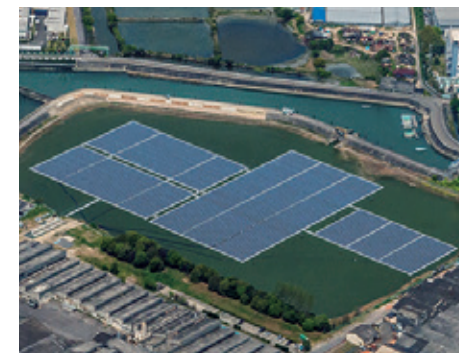
Water floating solar power generation plant (Kinuura Plant)
