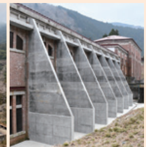
Reinforcement with buttress walls
