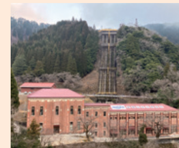
Higashi-Yokoyama Hydroelectric Power Plant after completion of reinforcement work
