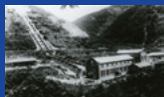
1 Nishi-Yokoyama Power Plant (1916-1963)
