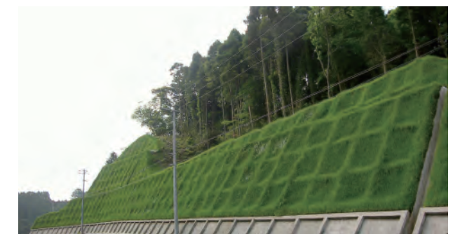
Slope constructed using the GT frame®
