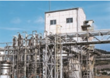
LiPF 6 production facilities
