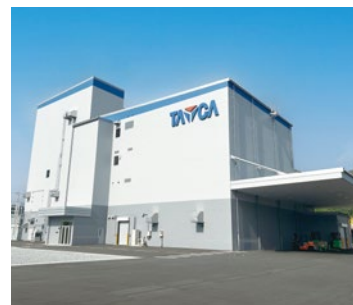
Exterior of Kumayama 4th. Plant
