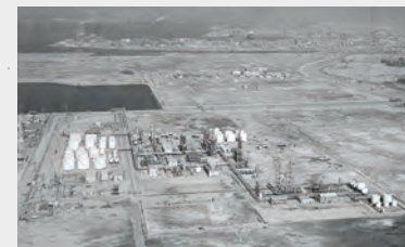
Nissan Petrochemicals Chiba Plant (1968)
