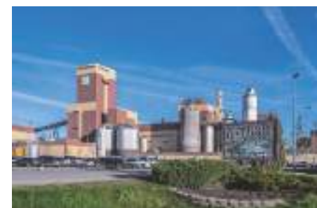
Alberta-Pacific Forest Industries Inc.の外観
