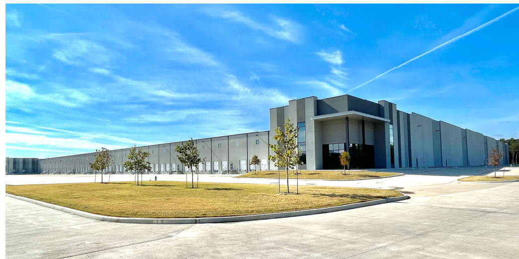
TOYO's new panel plant in the US
