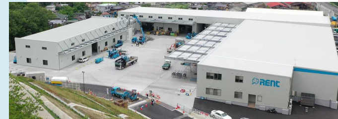
Maintenance Facility: RENT Nagoya Management Center
