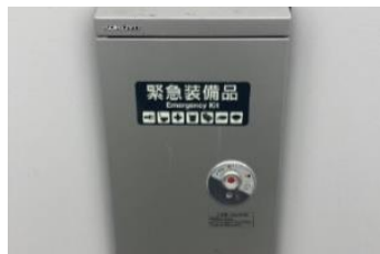
Installation of disaster supplies
