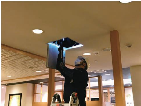
*A ceiling-space inspection using a 360° camera
