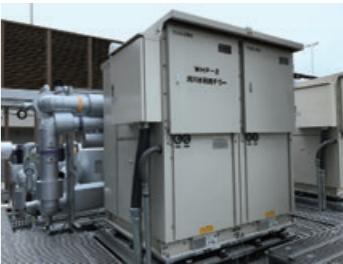
Heat pump that uses river water
