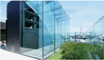
Natural ventilation (rooftop solar chimney)
