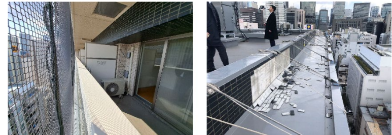
BEFORE The building was 18 years old and the tiles were peeling off badly, so netting had to be installed on the exterior walls to prevent accidents.
