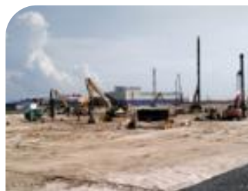
Construction site (as of June 2025)
