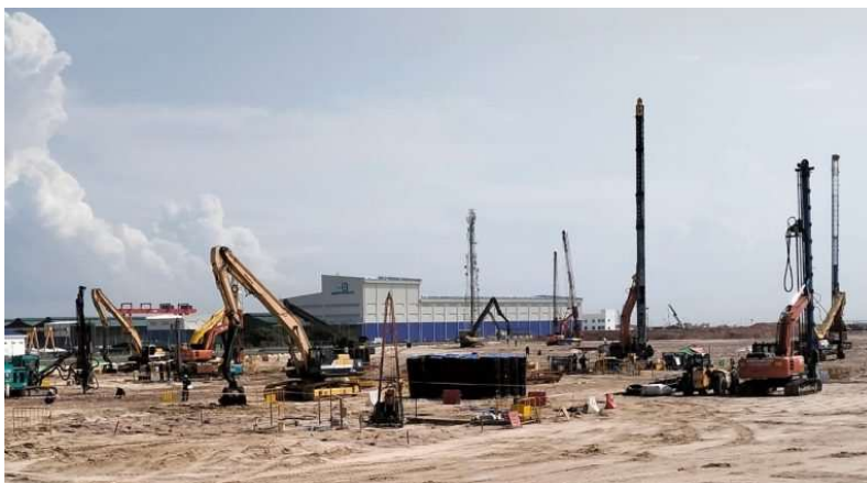
Construction site (as of June 2025)
