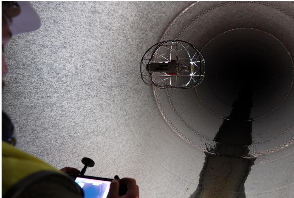
Safe and Efficient Pipeline Facility Inspections with the "ASIO X"
