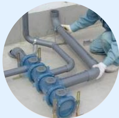
Equipment Installation (Plumbing, electrical wiring etc.)
