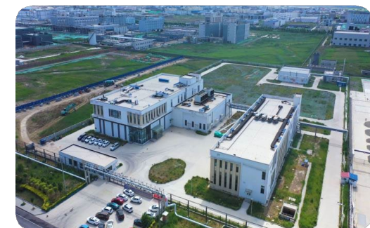
Active Pharmaceutical Ingredient (API) Facility (Cangzhou) Annual production capacity of 50 tons
