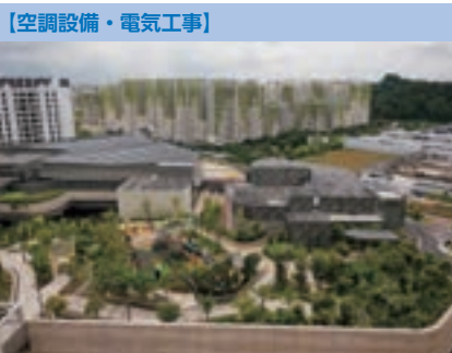
Housing and Development Tengah Park Centralised Cooling System (シンガポール)
