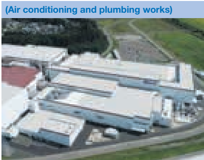
Nipro Corporation Odate Factory No. 7 (Akita Prefecture)
