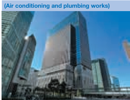
JP Tower Osaka (Osaka Prefecture)
