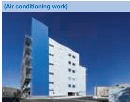
NRT12 Data Center (Implementation) (Chiba Prefecture)
