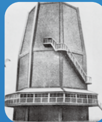
First domestically-produced cooling tower
