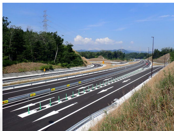
Pavement work on Onahama Road in Yamada
