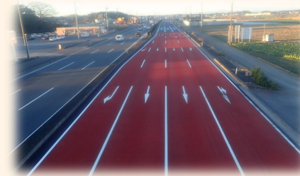
Surface repair work within jurisdiction of Kokubunji Branch Office <Strongphalt, a highly durable asphalt mixture>
