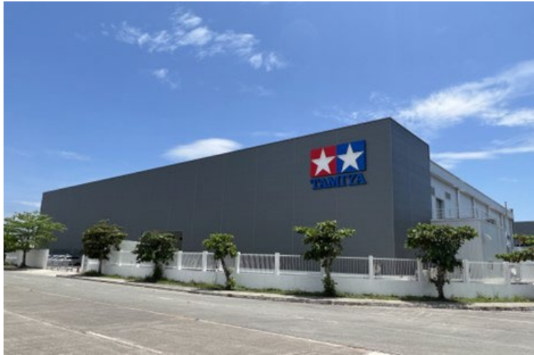
TAMIYA Philippines, Inc. New Factory Building
