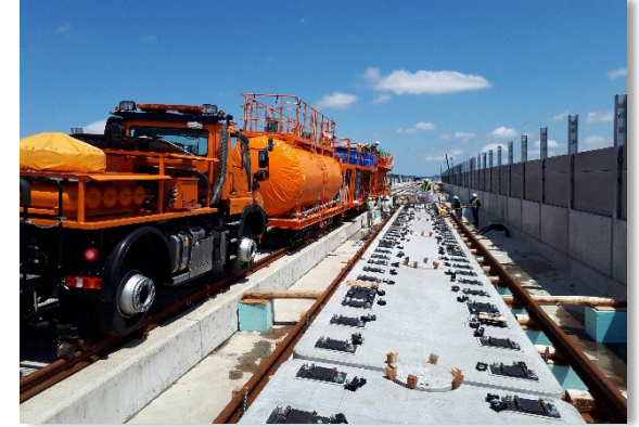
Hokuriku Shinkansen Fukui track construction
