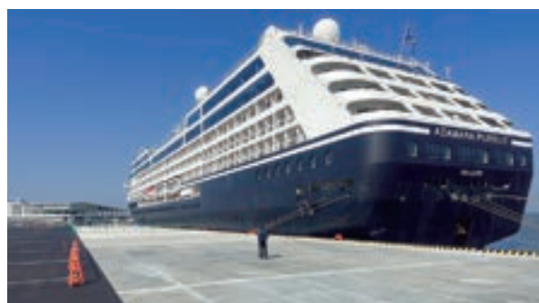
Kanazawa Port Cruise Terminal restored using PRC slabs
