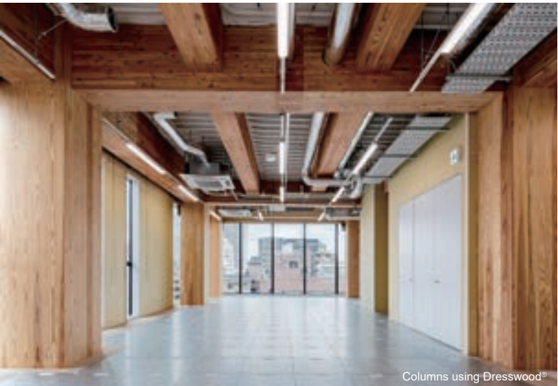
Columns using Dresswood®
