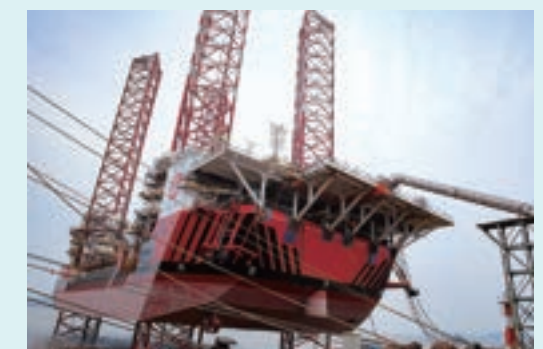
JWFC SUNRISE under construction in Shanghai
