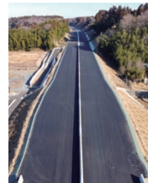
Higashi-Kanto Expressway Togasaki Construction Customer: East Nippon Expressway Company Limited, Kanto Branch
