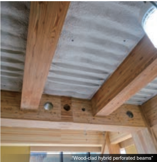
"Wood-clad hybrid perforated beams"
