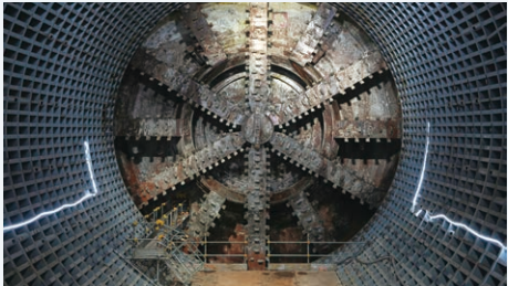
Yokohama Shonan Road Tunnel construction Phase 3
