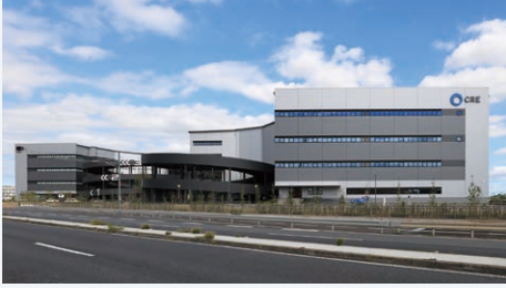
New construction of LogiSquare Fujimino A & B
