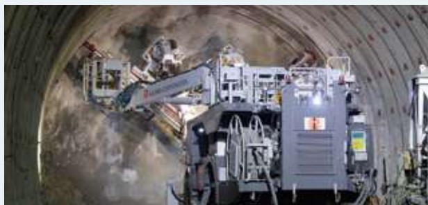
A4CSEL for Tunnel, automated rock bolt installation
