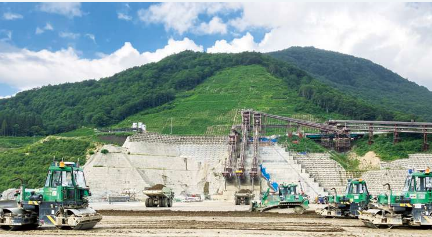
A 4 CSEL*-guided automated construction machinery building an embankment at Naruse Dam (August 2023)
