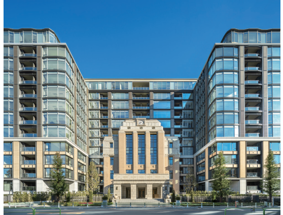
Minato-ku Mita 1-chome Project (tentative name) (Minato-ku, Tokyo) Owner: Mitsui Fudosan Residential Co., Ltd. Mitsubishi Estate Residence Co., Ltd.
