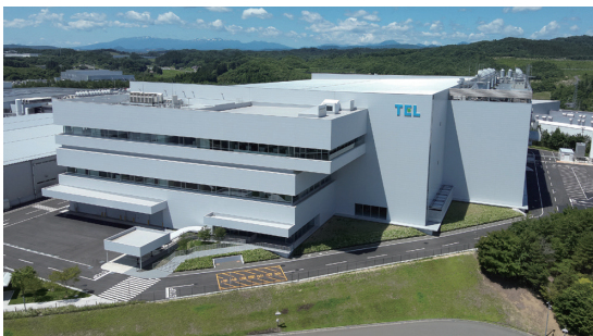
Tokyo Electron Miyagi Ltd. New Building Construction Work for Development R&D Building 3 (Kurokawa-gun, Miyagi) Owner: Tokyo Electron Miyagi Ltd.
