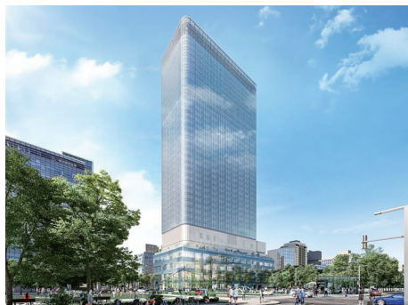
Odori-nishi 4 South, Type 1 District Redevelopment Project (Sapporo-shi, Hokkaido) Owner: Odori-nishi 4 South District Urban Redevelopment Association
