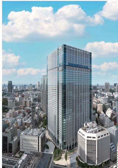
Newly Building Construction Work for Akasaka 2-chome Project (tentative name) (Minato-ku, Tokyo) Owner: Mori Trust Co., Ltd. NTT Urban Development Corporation
