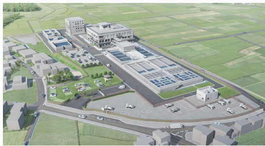
Kabutoyama Water Treatment Plant Upgrade Project, Construction of New Water Treatment Plant (Himeji-shi, Hyogo) Owner: Himeji City
