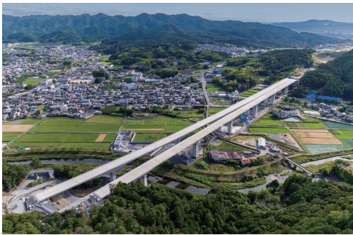
Shin-Meishin Expressway, Construction Work for Ujitawara No. 2 Viaduct (PC superstructure) (Tsuzuki-gun, Kyoto) Owner: West Nippon Expressway Company Limited
