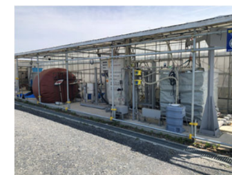
Pilot-scale methane fermentation system
