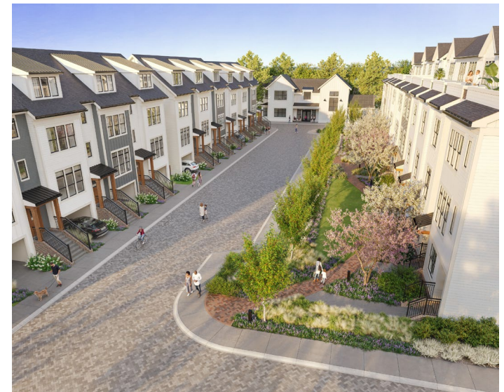
▲ “Elm Hill Townhouse” project State of North Carolina
