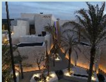
Expo 2025 Osaka, Kansai, Saudi Arabia Pavilion Construction Site: Osaka Prefecture
