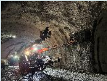
Tokai-Hokuriku Expressway (4 Lane Expansion), Tsubakihara Tunnel Construction Construction Site: Gifu Prefecture
