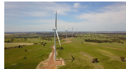
Flat Rock Onshore Wind (Potentia Energy)
