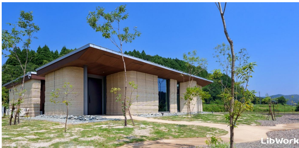
Lib Earth House Model B was built with 3D printing technology.
