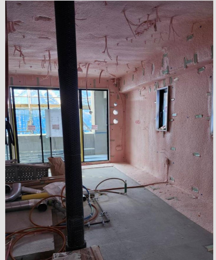
Replaced by products such as Aqua Foam NEO (on-site foamed urethan)
