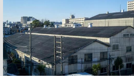
Factories of major building materials manufacturers
