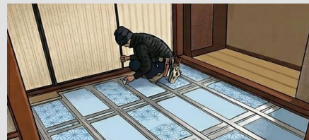
Floor insulation in Single-Family Homes (XPS boards)
